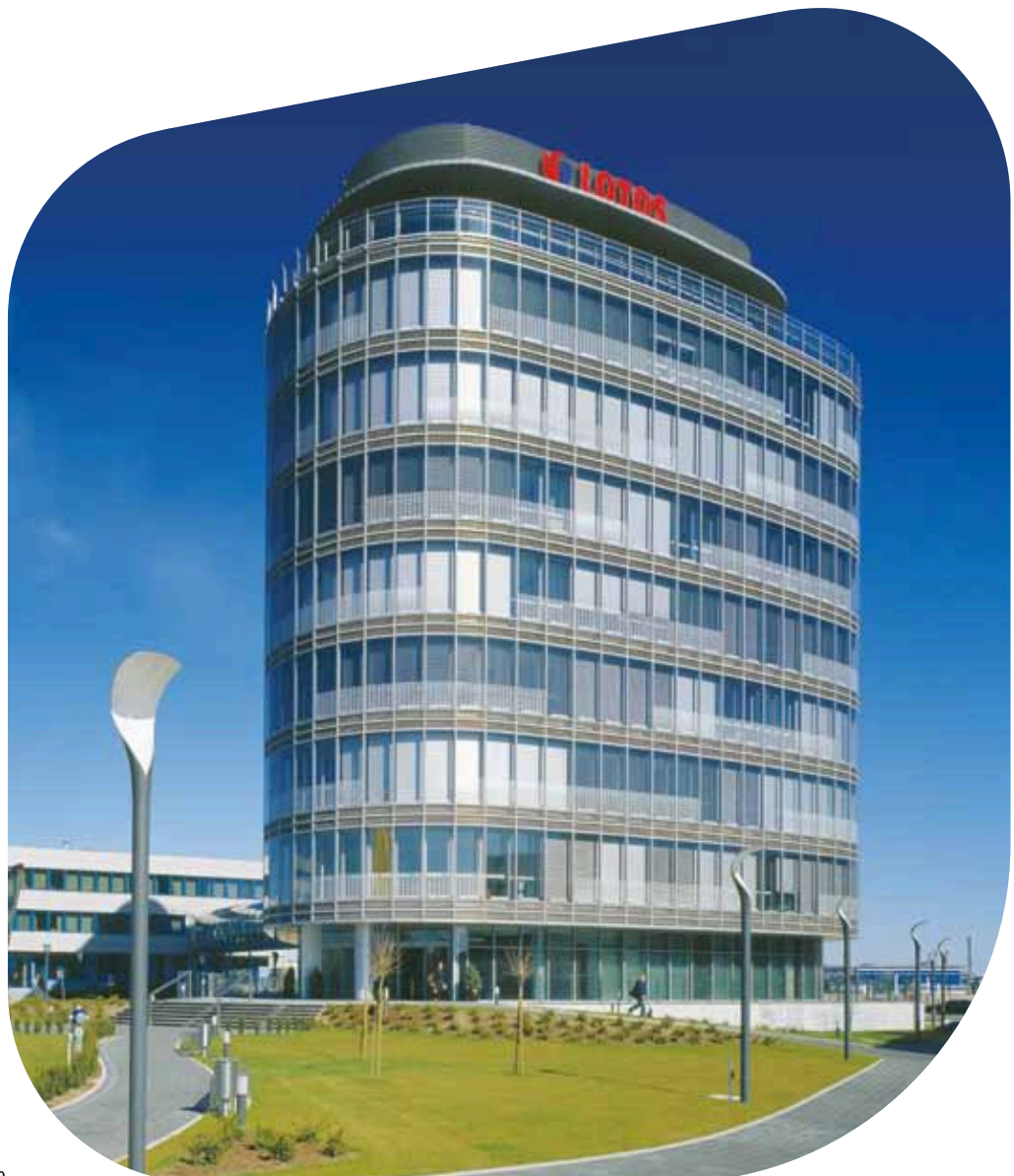
Lotos SA office building, Gdańsk, Poland – Pilkington Suncool™ 70/40
